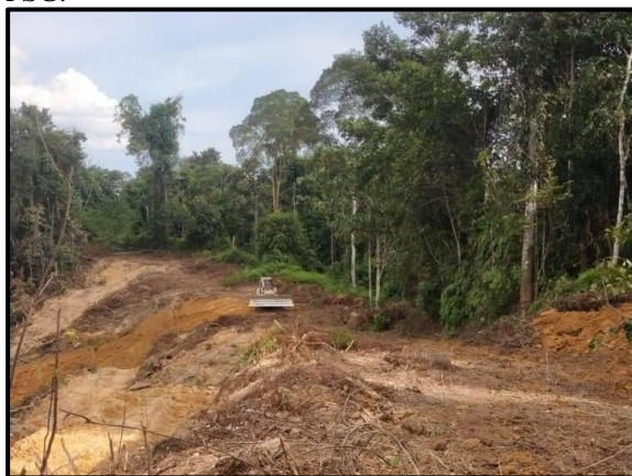
Gambar 2. Proses Land Clearing PT PSG (PT PSG, 2020)
