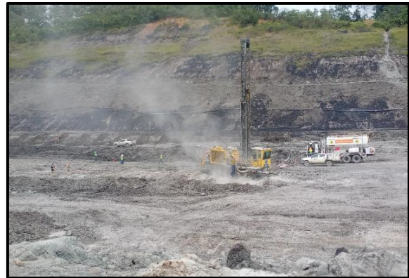
Gambar 3. Proses Drilling Hanwa Mining Services
