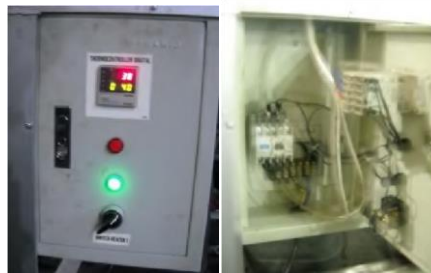
Figure 14. Temperature control systemat Single Stage Compressive Test
