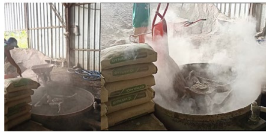
Figure 2. Mixing area of UD. TGM
